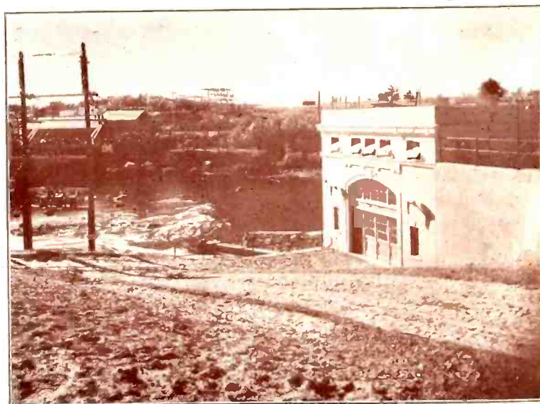
CENTRAL MAIN POWER CO. ON ANDROSCOGGIN RIVER ABOVE LEWISTON
