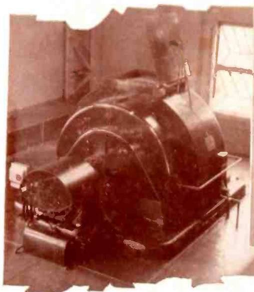
A Lux-protected Synchronous Condenser in the Trenton Switching Station of the Public Service Electric and Gas Company of New Jersey.
