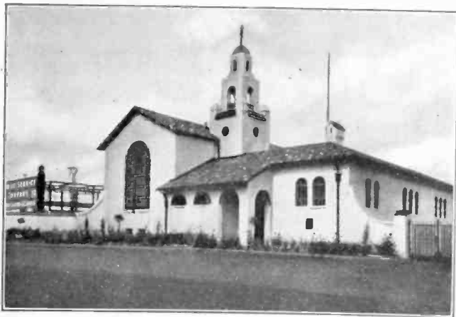
FIG. 8—VOLLMER ROAD SUBSTATION
