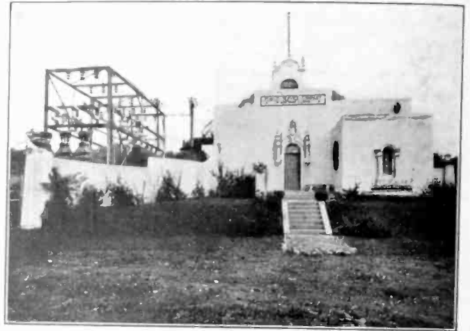
FIG. 9—GLEN ELLYN SUBSTATION
