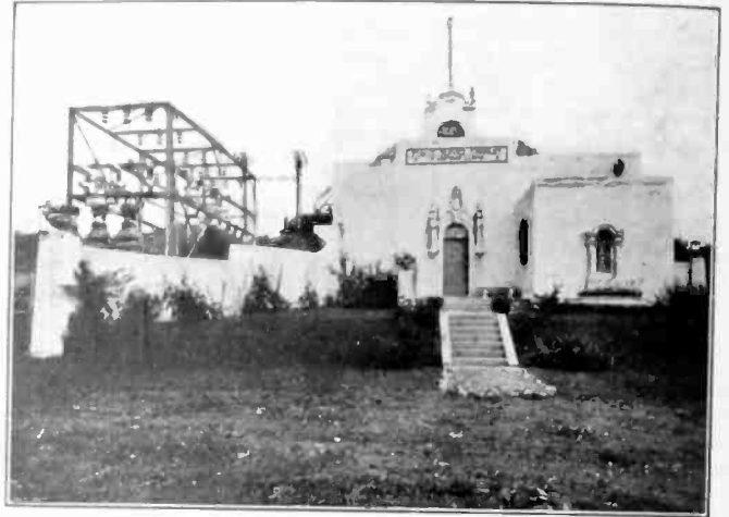
FIG. 9—GLEN ELLYN SUBSTATION
