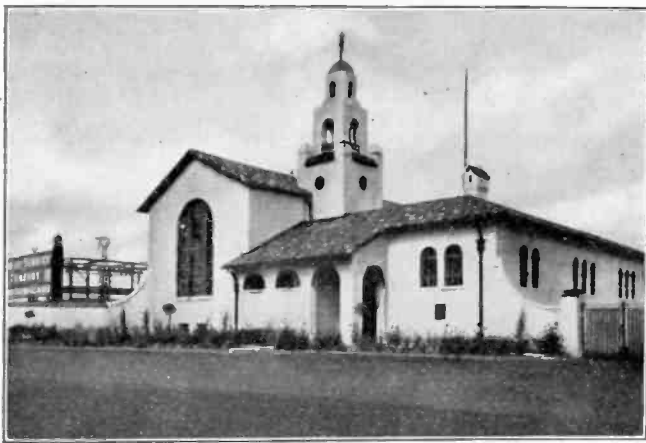
FIG. 8—VOLLMER ROAD SUBSTATION
