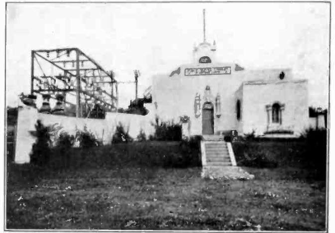
FIG. 9—GLEN ELLYN SUBSTATION
