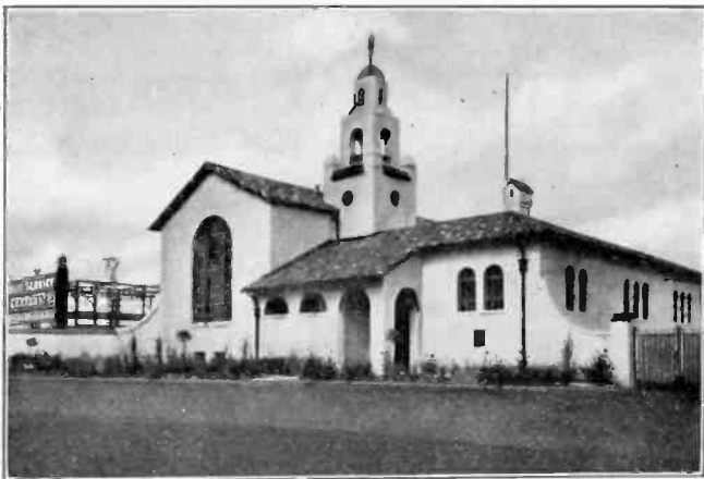
FIG. 8—VOLLMER ROAD SUBSTATION
