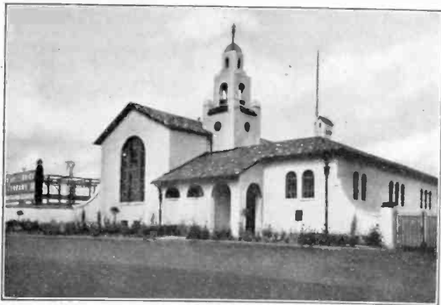
FIG. 8—VOLLMER ROAD SUBSTATION
