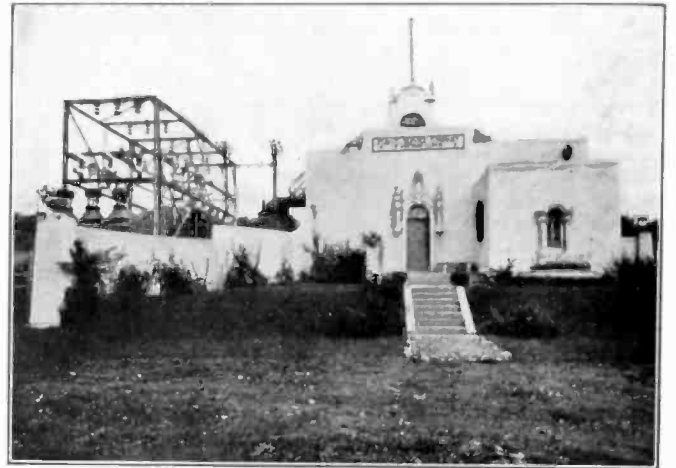
FIG. 9—GLEN ELLYN SUBSTATION
