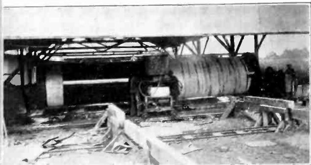
SPIRAL WRAPPING IN THE YARD
