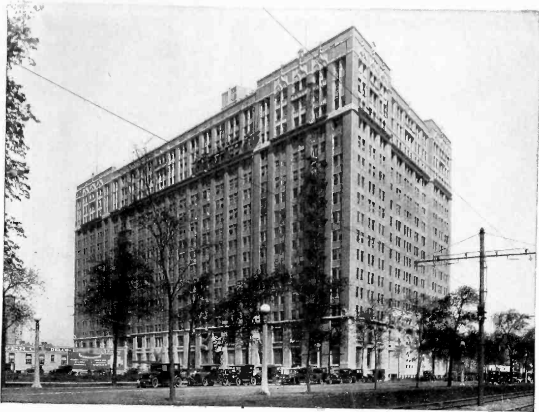
Furniture Mart, Chicago, Served by Kuhlman Transformers
