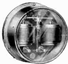
Typical D-C. Differential Relay
