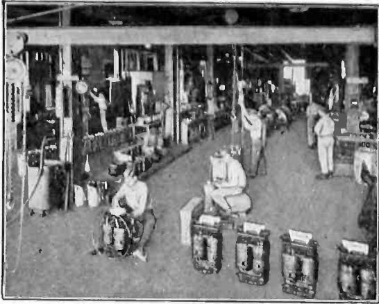
Small assembly floor where Type H. E. Transformers are assembled.
