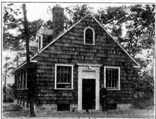
FIG. 23—RECEIVING STATION, RIVERHEAD, LONG ISLAND
