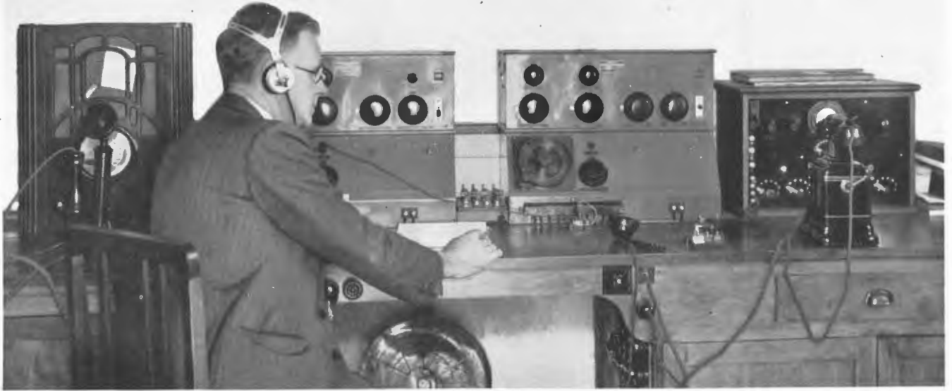
Interior D.F. Station at Essendon, Vic.
