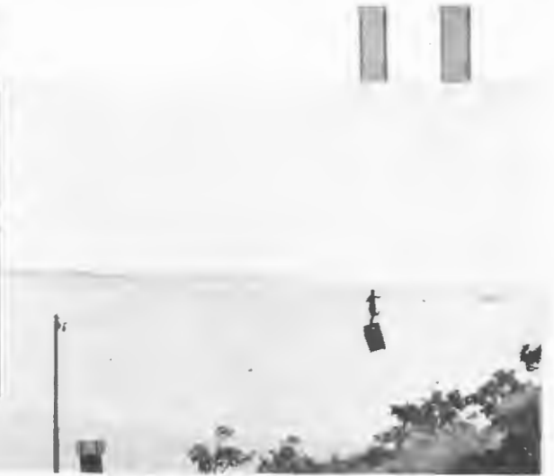
The extremely difficult path leading to the wireless station made the use of a "Flying Fox" a practical necessity. Portion of apparatus being transported.
