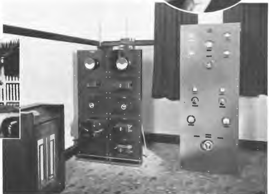
Portion of series modulated 50 watt transmitting equipment of 4WK, Warwick.
