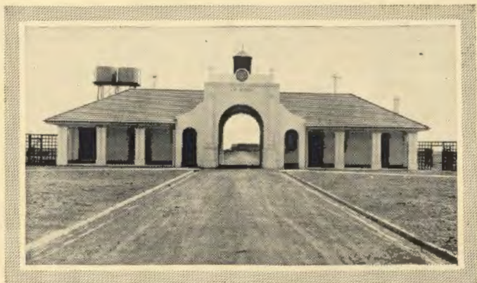
Position of Staff Quarters and Club House, Beam Wireless Station, Ballan, Victoria.
