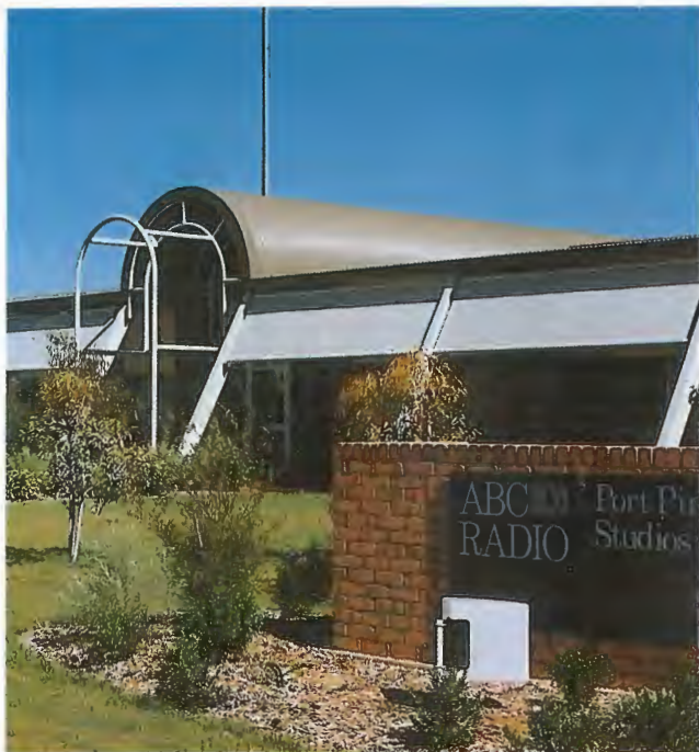
The new building
