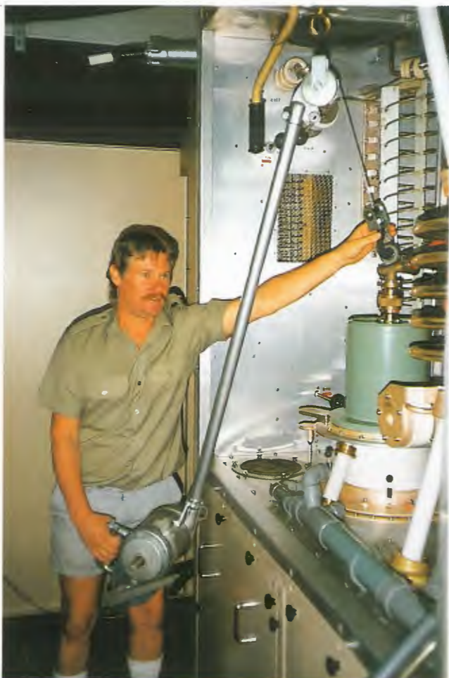
Gordon Hall about to lift Thomson TH573 tube Radio Australia Carnarvon.
