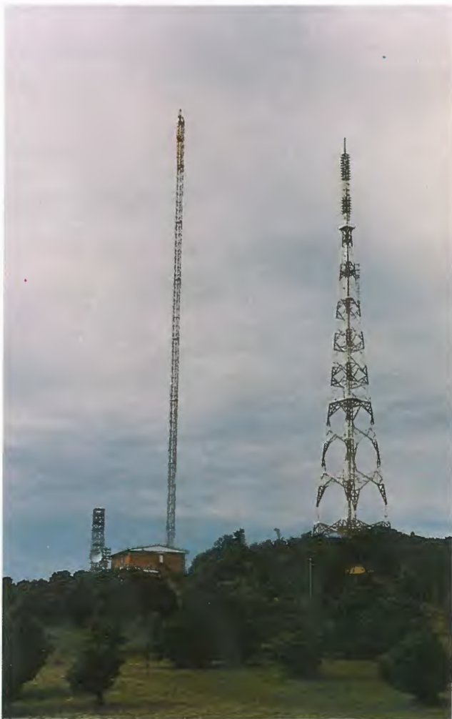
Newly erected mast alongside original tower.
