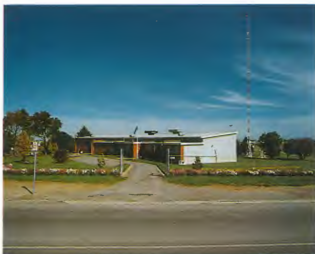
5AN building and mast.
