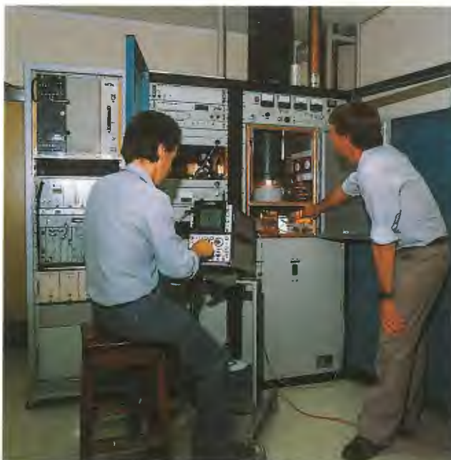
Peter Usher (L) and Martin Morris adjusting 20kW NEC FM transmitter.
