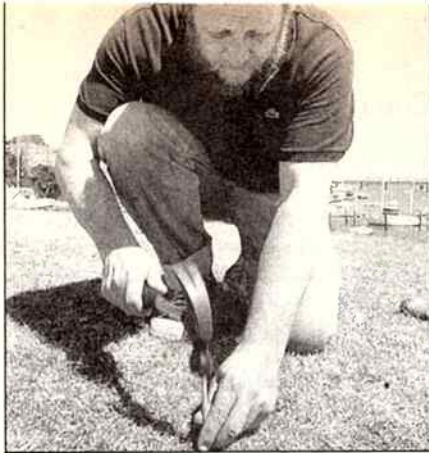
Measure out a square on the ground, the size of the element you're building. Hammer short pegs into the ground to mark the corners.
