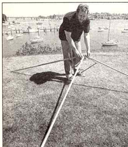
Lay the completed 'spider' over the pegged-out square. The corner pegs will indicate where to drill the spreaders.
