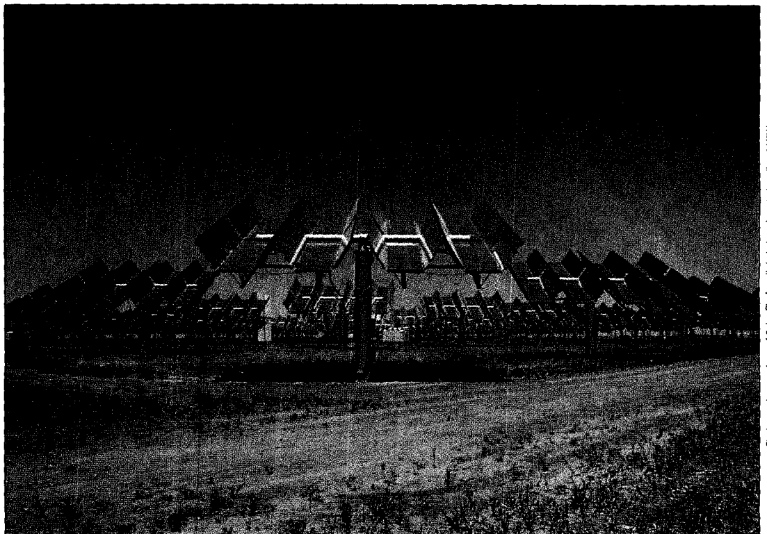
World's largest photovoltaic installation (6.5 megawatt) at Carrisa Plains, California.
