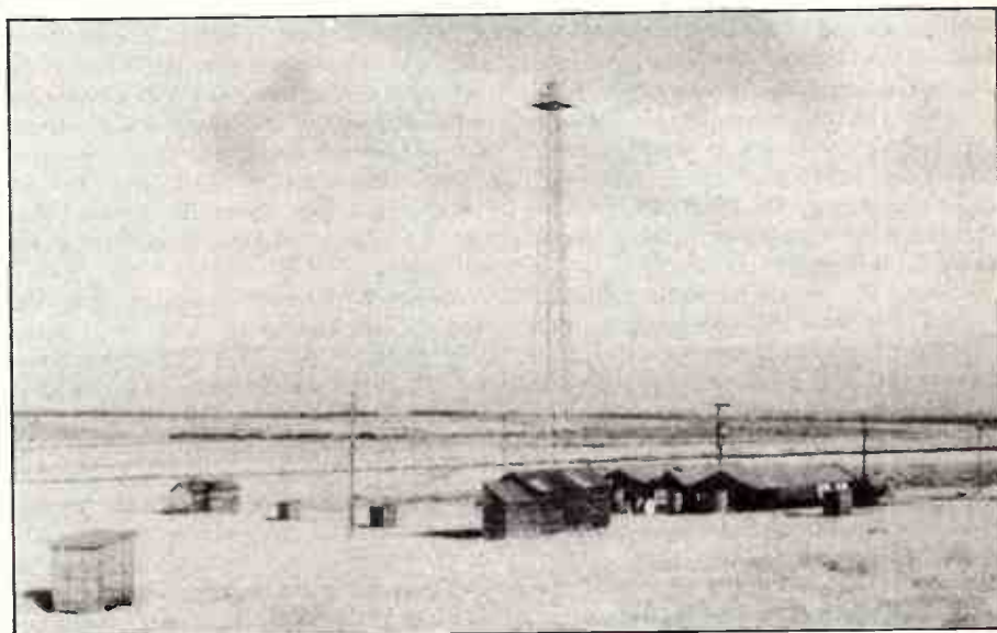
The detectors near the centre of the Haverah Park shower array in England. The scintillators are housed in small wooden huts around the central laboratory building. (Photo by Mark Lawrence, Leeds University.)
