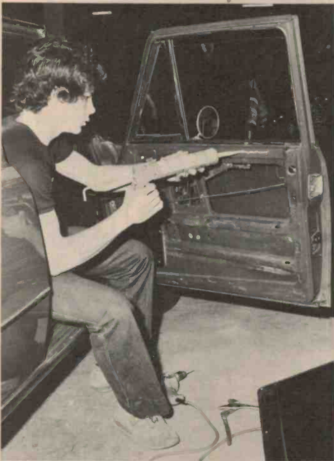
It is important to seal the door cavity as much as possible, particularly around the inside trim. Silastic is recommended for this job.
