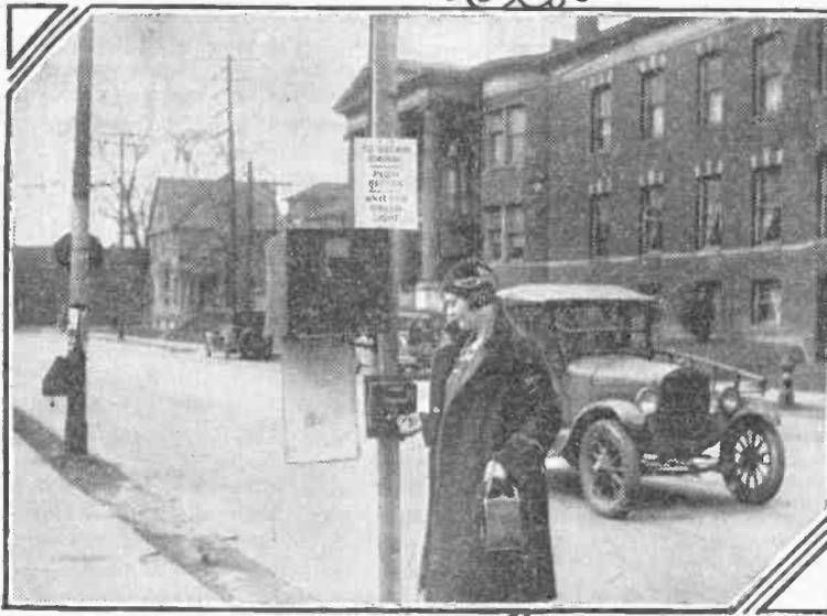
Automatic Traffic Signal. A recently installed automatic traffic device, which operates by sound wave. Light stays red until driver signals with horn that he is ready to cross. The impulse of the signal changes the light to green for 30 seconds. Pedestrians operate the signal by button.
