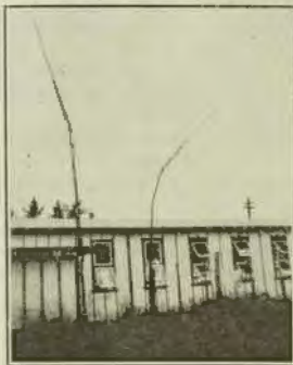
Radio Hill is the name of the prominence upon which the new transmitting station for 7ZL is being built outside Hobart.
