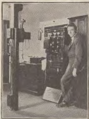
The control room at 4QG.
