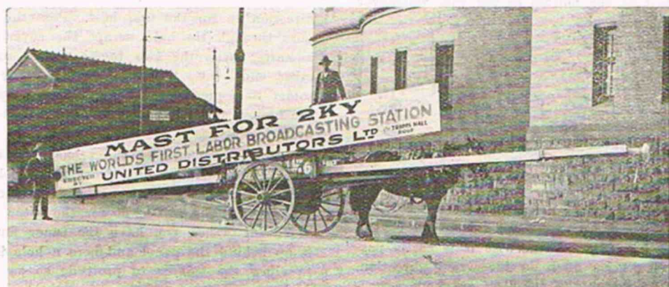
The Mast being conveyed to the new Station
