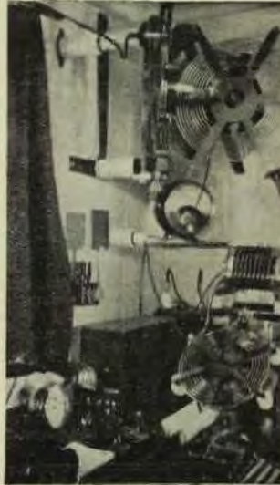
The Bakara's Wireless Installation.
