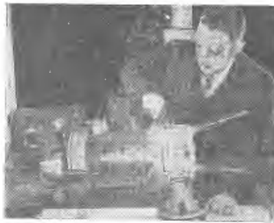
Fig. 6.—Resnatron tube delivers 50 kW at Microwave frequencies. It may be applied to Microwave heating.
