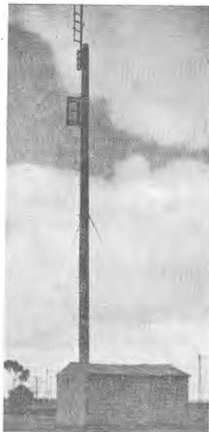
View of the MTR slave station used in trials on Sydney-Melbourne air route. The main transmitter aerial is at the top of the wooden mast and the slave receiving aerial below it.
