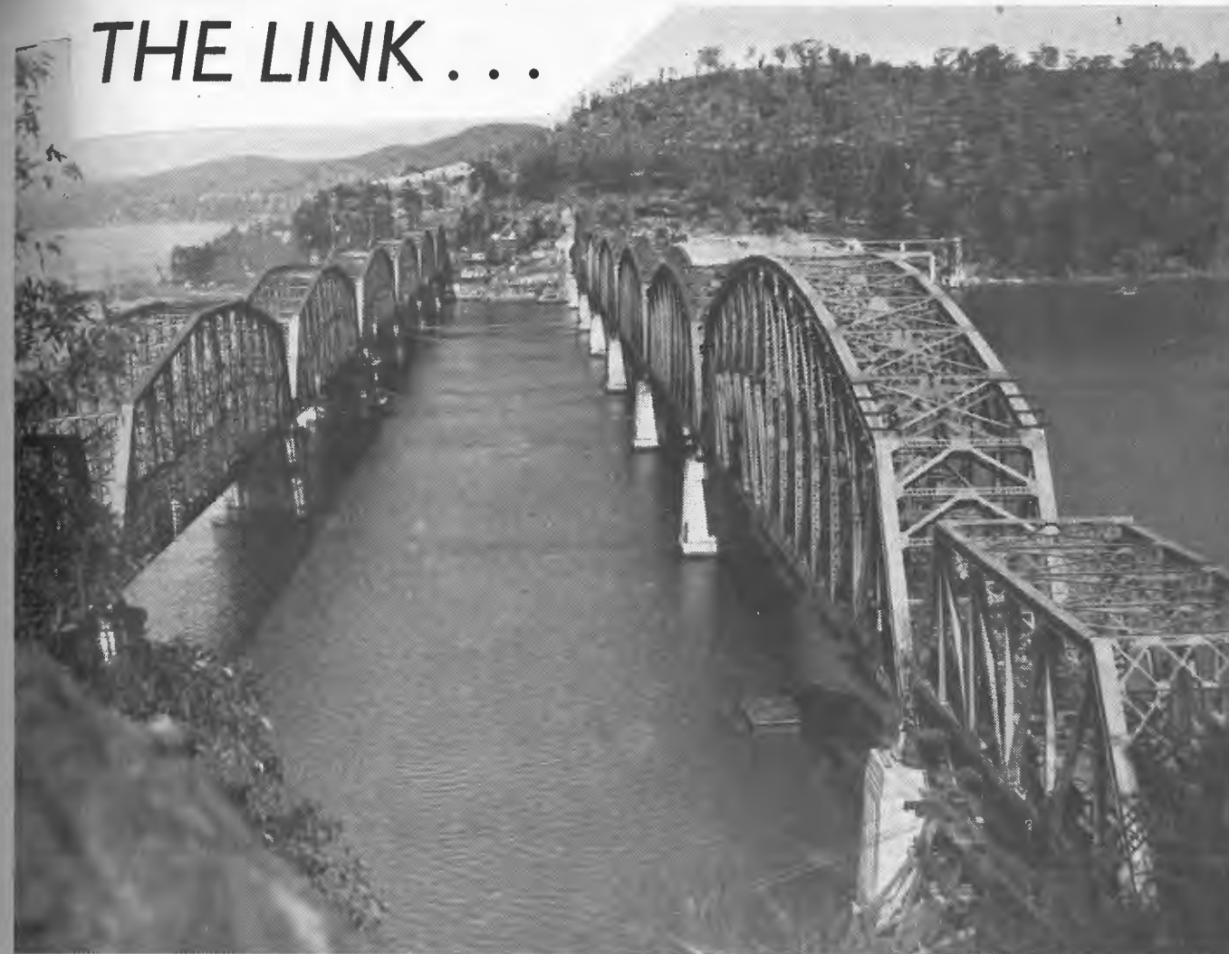
OLD AND NEW HAWKESBURY RIVER BRIDGES
