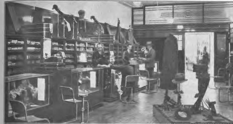
Modern headquarters store of Wardrop, Tailors, of Melbourne.
