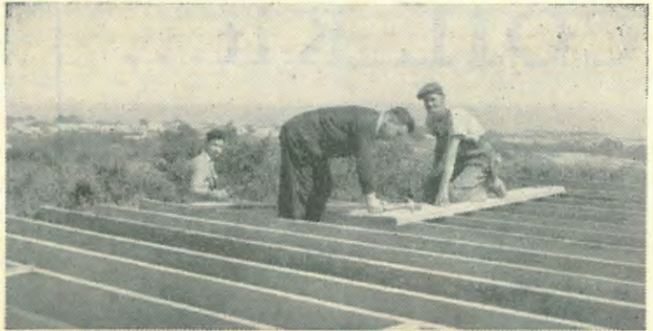
Mr. Hull lends a hand on the attic floor joists of the new home for "Australasian Radio World." Over the tree tops in the background can be seen the town of Mornington, with the Bay beyond.
