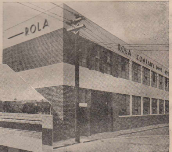
RIGHT: Threequarter front view of the Rola factory recently completed at Richmond, Melbourne.
