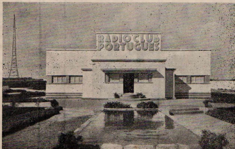
This building houses the broadcast and shortwave transmitters of stations operated by members of the Portuguese Radio Club.
