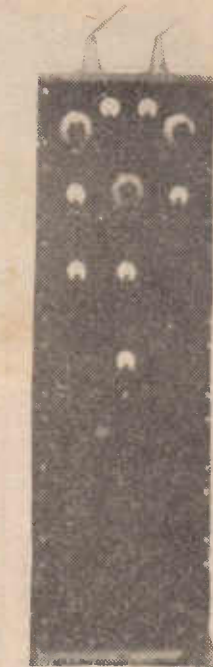
★ The neat rack and panel transmitter assembly at VK2TI.
