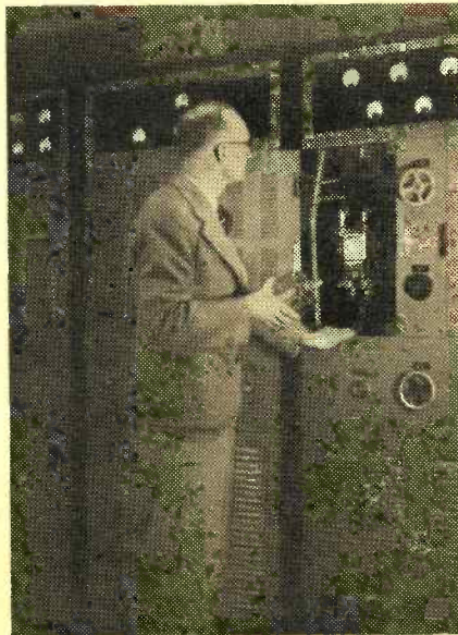
● Chief Technician Bert Sctrine (VK3BI) holding one of the 833 Class B modulators at the transmitter.
