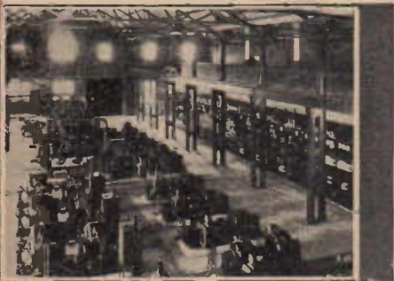
Power generating plant at the Beam Wireless Station, Ballan, Victoria.
