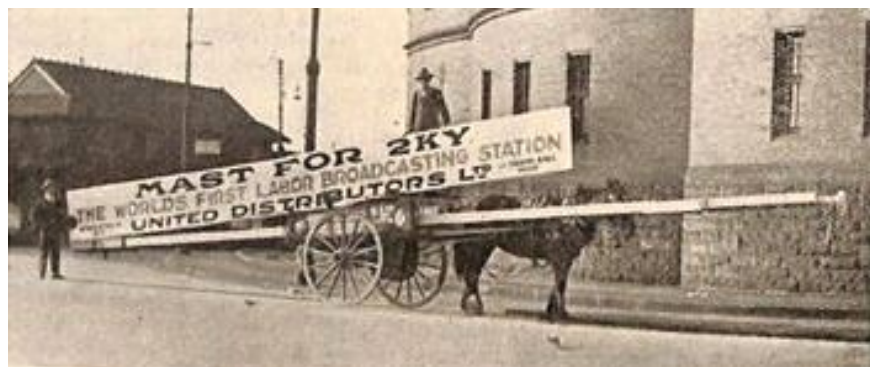
2KY TOWER ON ITS WAY TO BE INSTALLED
