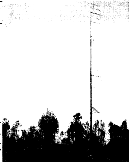
Gympie ARC repeater site. On the tower are two 2 metre and two 70cm antennas plus a solar panel which is used to power the repeaters. See story page 46.
