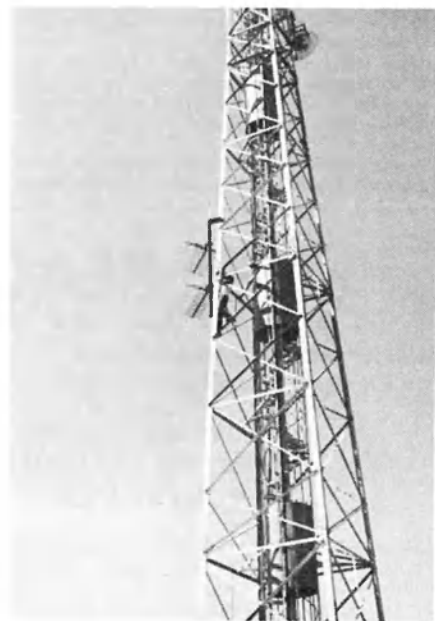
The corner reflectors being raised up the collimation tower. Various other NASA antennae is on the tower and the channel 6 repeater VK1RAC antenna is at the very top.
