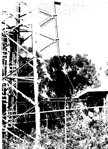
The Corner Reflectors being raised up the Collimation Tower.
