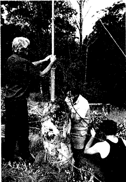
John VK4ZDV, Aaron VK4AHO and Grant VK4KJR/P29KJR erect a pneumatic mast on loan from the State Emergency Services for the second WICEN repeater antenna. (See page 14 for cover story.)
