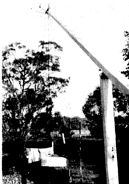
Picture 1: Pole on footing partially raised.
