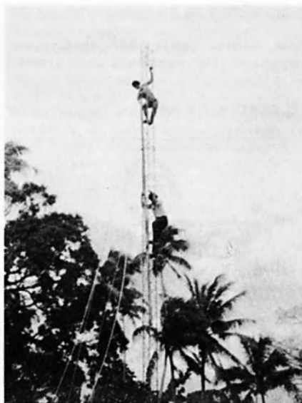
Erecting the tower which came from the T and T Department for a nominal fee.
