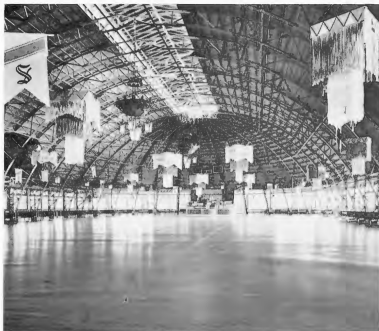
Above is shown part of the Saltair Dance Pavilion, largest dance floor in the world, at Saltair, Utah, which suffered from poor acoustics until Radio Sound & Service, Inc., of Salt Lake City, corrected the acoustics—and made a nice profit—by installing a complete RCA Sound System.
