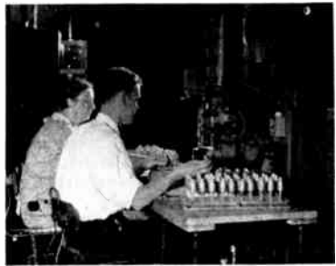
Welding Metal Tubes
