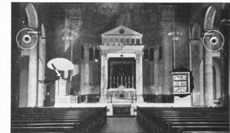
Interior of St. Gregory's Church, Brooklyn, showing the RCA sound system units that solved a difficult problem of poor acoustics.
