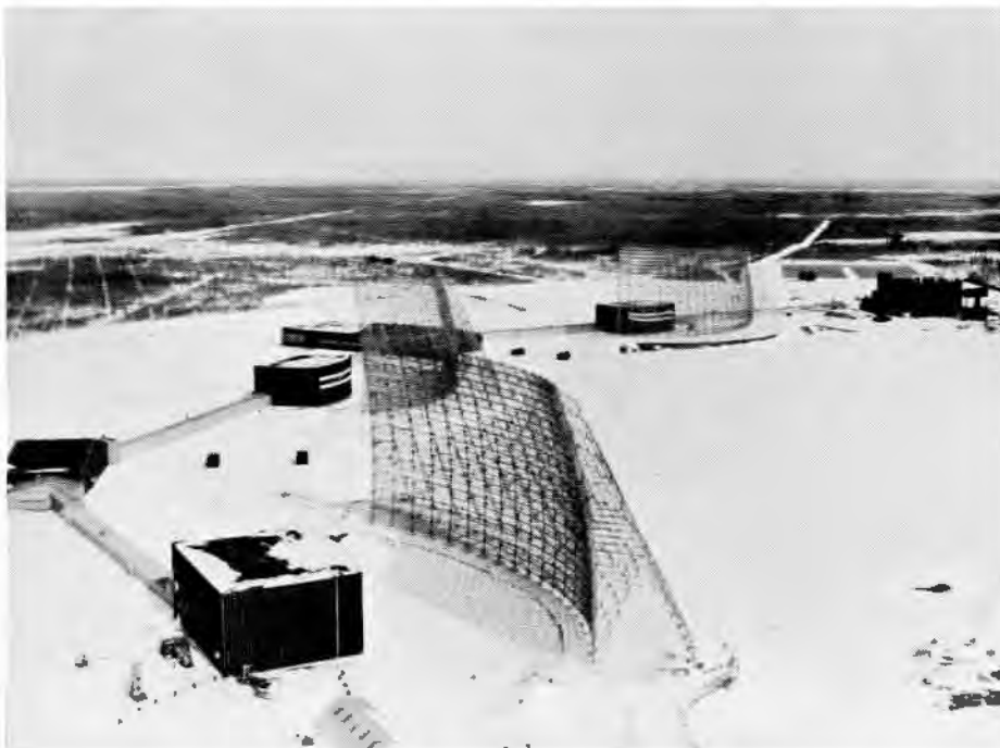
BMEWS Site II with three detection radars and scanner buildings.
