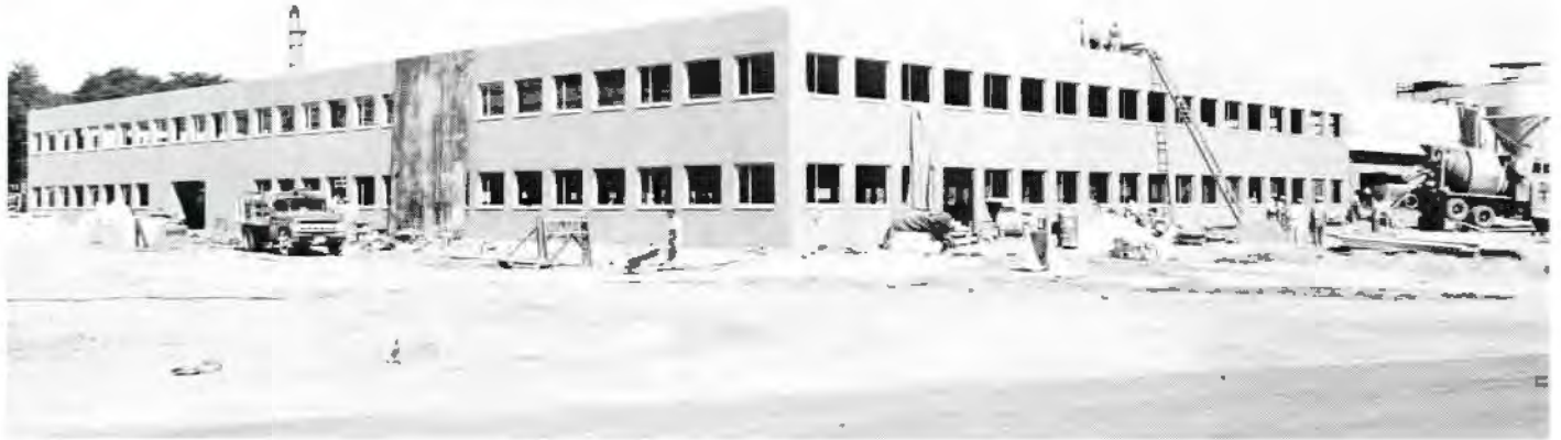
This progress photo shows Cherry Hill's new addition as it looked on July 15th.
