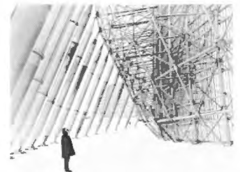
Huge stanchions support the radar antennas.
