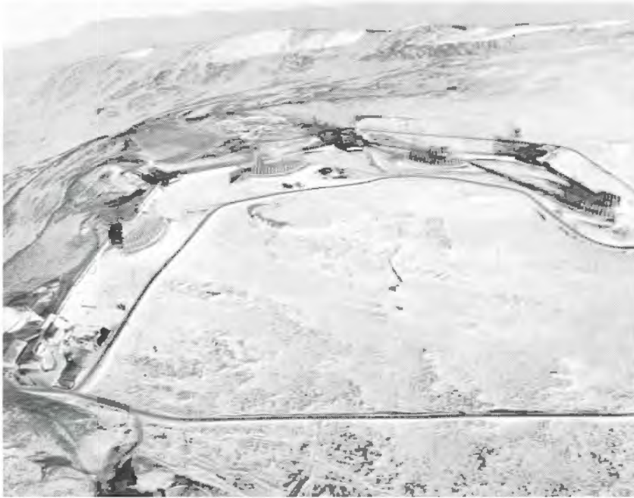
This is BMEWS Site I, Thule, Greenland, casting its shadow over the Wolstenholme fjord. Each antenna is 400 feet long and 165 feet high.
