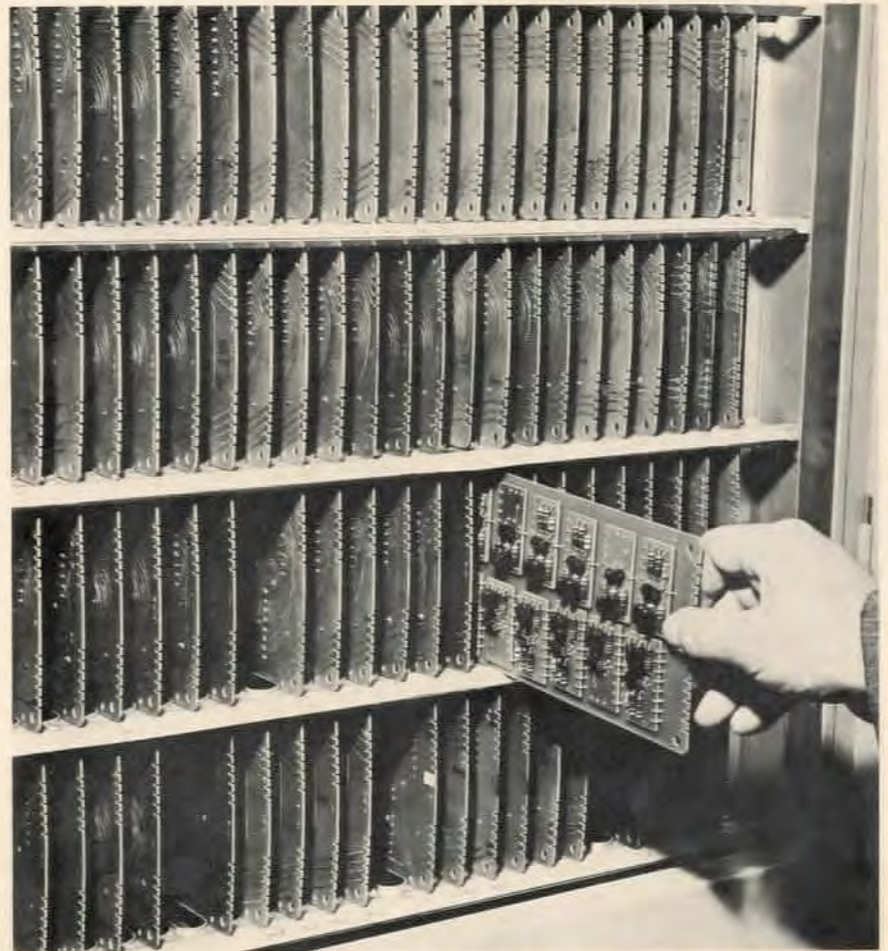
The plug-in assembly is installed in the system simply by sliding it into position. The assembly takes up only \frac{1}{4} the space required by vacuum tube circuitry of the same capacity.
