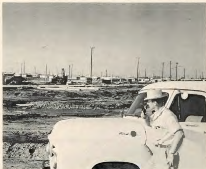
Superintendent of the Larwin Construction Company radios his report to headquarters from one of three building sites.
