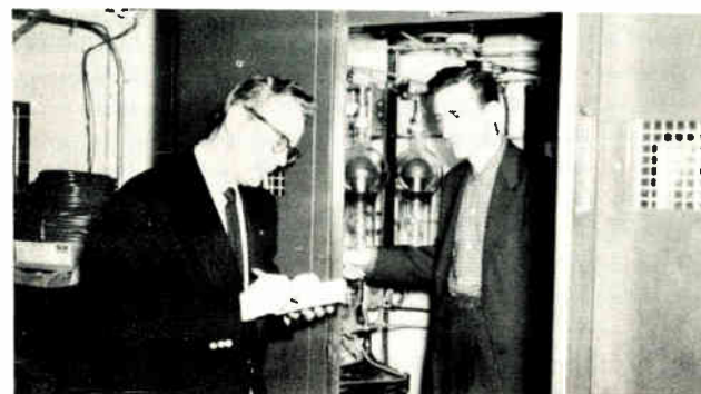
Checking the performance of the powerful TV transmitter, Lou takes notes as Jack makes adjustments
