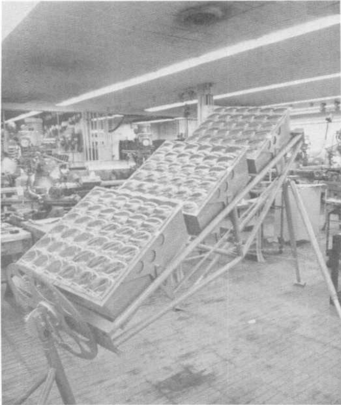
Fig. 21—Experimental 100-W photovoltaic generator.
