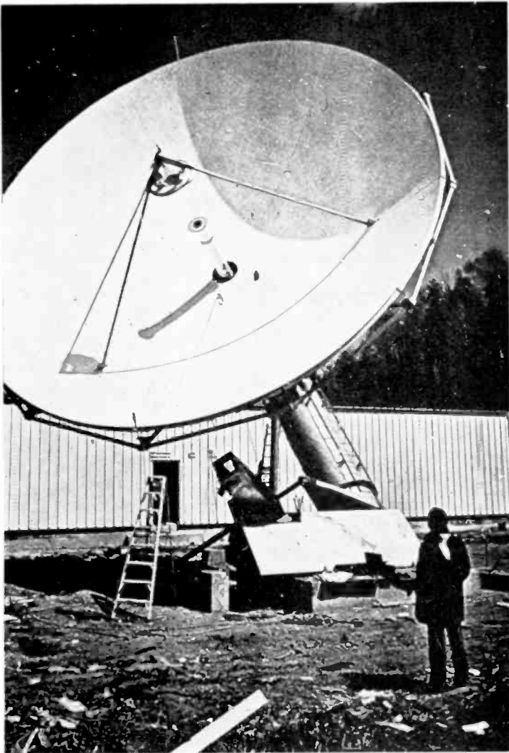
Fig. 2—Antenna system mounted on an hour-angle declination pedestal.
