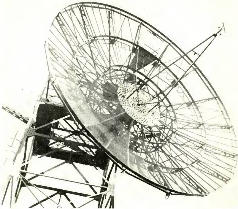
Fig. 17—Paraboloid antenna 40 feet in diameter at radiation laboratory on Covey Hill, Quebec, completed in May 1954.
