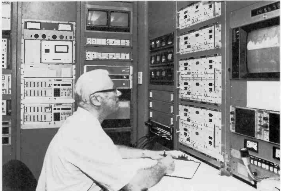
Fig. 6. Microwave receiver and transmitter control room. The operator controls all microwave receivers along with the main broadcast transmitters.
