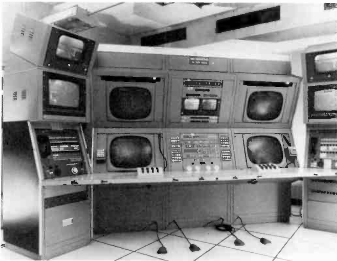
Fig. 2. The Range Safety Display System provides Air Force Range Safety Officers with accurate electronic displays of Space Shuttle and other launch-vehicle flight conditions, plus the ability to remotely control transmitters that can send destruct signals if necessary. MTP provides maintenance and software services.
