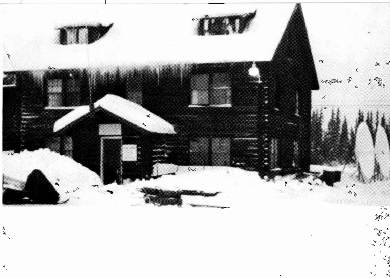
Fig. 2 Telemedicine by satellite experiments in Alaska began in 1974. The two antenna dishes here link the lone nurse at the Alaska Area Native Health Service Clinic at Ft. Yukon with physicians at an Anchorage hospital.
