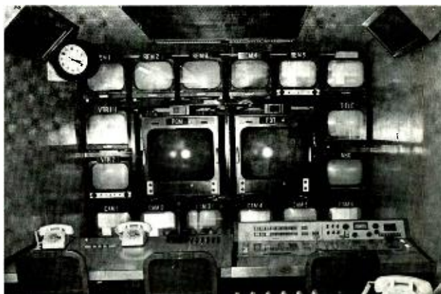
Fig. 7—Photo monitors and console.
