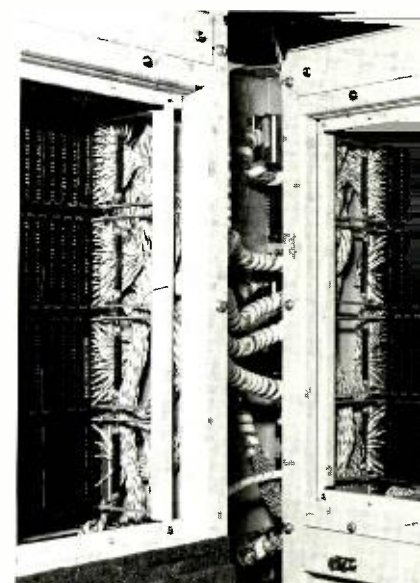
Fig. 6—Typical interconnecting cable harness between platter frames.
