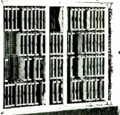
Fig. 4a—Platter mounted with plug-in boards in position.
