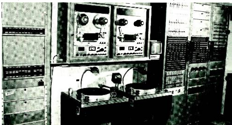
Fig. 2—Associated turntables, tape recorders, and cabinet racks containing amplifiers.
