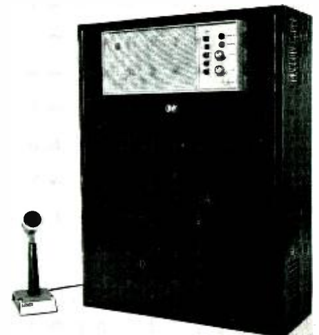
Fig. 11—Typical controlfone equipment in outdoor type cabinet housing.
