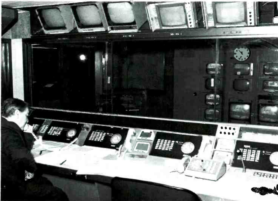
Fig. 2 — The Executive Deck is adjacent to the BOC area. This is used as a coordination area for the Studio 5N (ad-lib) Production Control Room. Communication facilities provided for the Executive Deck are of the same type as those provided for BOC; however, no patchfield is provided. A number of loudspeaker panels (shown on the upper turret) are capable of assignment by the transmission center to amplify any of twenty incoming lines. This system is an NBC program monitoring system, not concerned with Telephone Company equipment.
