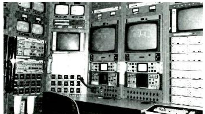
Fig. 4 (above) — Special test equipment is integrated into the transmission center. The signals generated by the test equipment include full-field color bar, window-modulated step, multiburst and grating; as well as \sin^2 vertical-interval test signals (VITS), and the vertical interval reference signal (VIR). Fig. 5 (below) — Character generator keyboard is centrally located within transmission.
