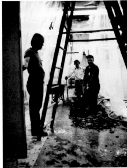
The incision—start of the trench used for the acid drain piping.
