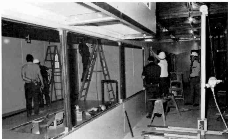
Furnace wall during construction.
