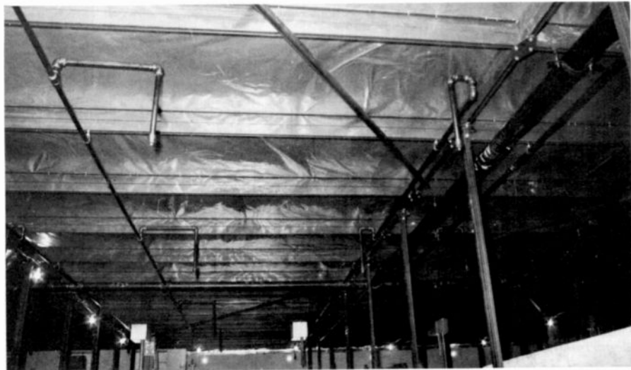
Underside of ceiling showing vapor barrier.
