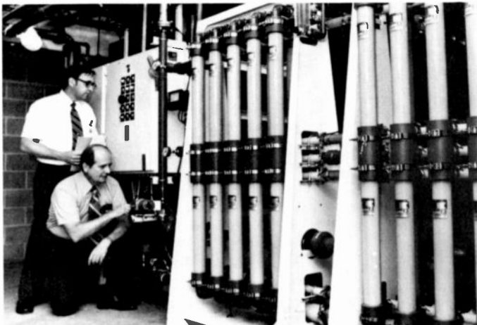
Tom Edwards (left) and Bob Blazek inspecting the new Ultra Filtration water system at Lancaster.
