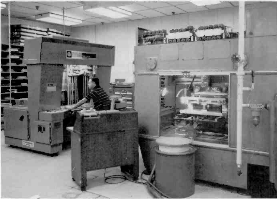
Fig. 5 — Automatic wire-wrapping equipment.
