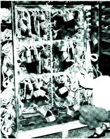
Bob McLaughlin in the Mechanical Packaging Engineering Lab setting up life tests on switches. The carousel-type tester in the foreground was developed in this Laboratory.
