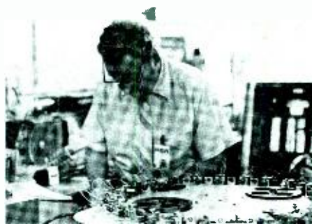
Bob McLaughlin in the Mechanical Packaging Engineering Lab setting up life tests on switches. The carousel-type tester in the foreground was developed in this Laboratory.
