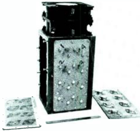
Fig. 3—Transpiration cooler with boxer fan.
